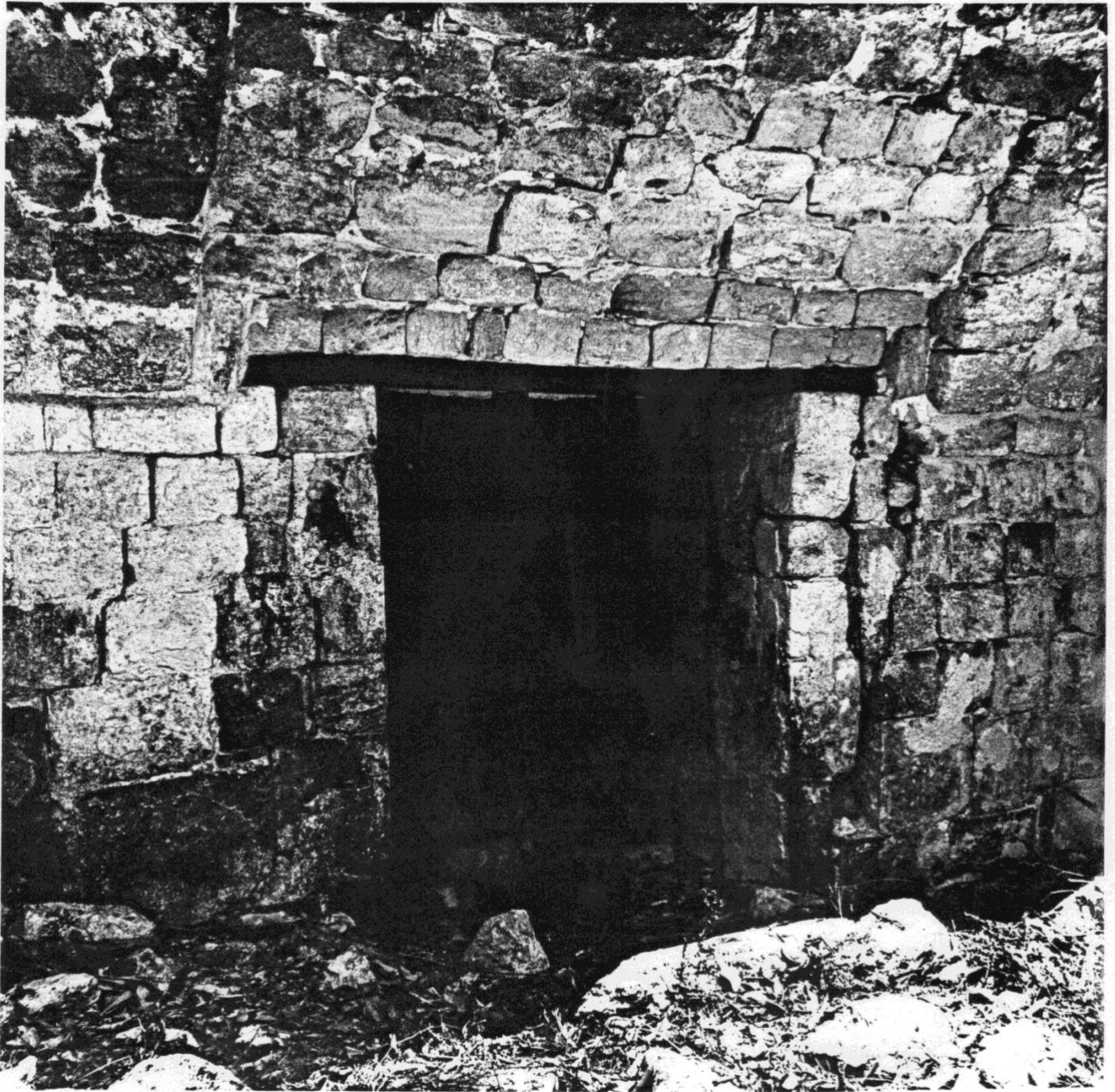
Fig. 8. Santa Rosa Xtampak, Main Palace, east side, probably Room 6. These planks are so well preserved that the stress has transferred to the jambs, causing them to sheer away from the wall. In this instance the jambs will buckle out before the lintels rot or break causing far more destruction than if the lintels alone broke.
