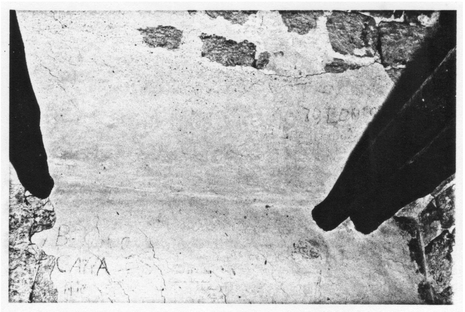
Fig. 3. Detail of the three wall beams in Room 8, looking west. The plaster is as remarkably preserved as are the three round beams. Since the wood is still flush to the pole this means these have not shrunk at all, quite a difference from the door lintels. Is that because a plank exposes more surface or because the poles have all the core intact and less surface area? Santa Rosa Xtampak, Main Palace, first floor, east side.
