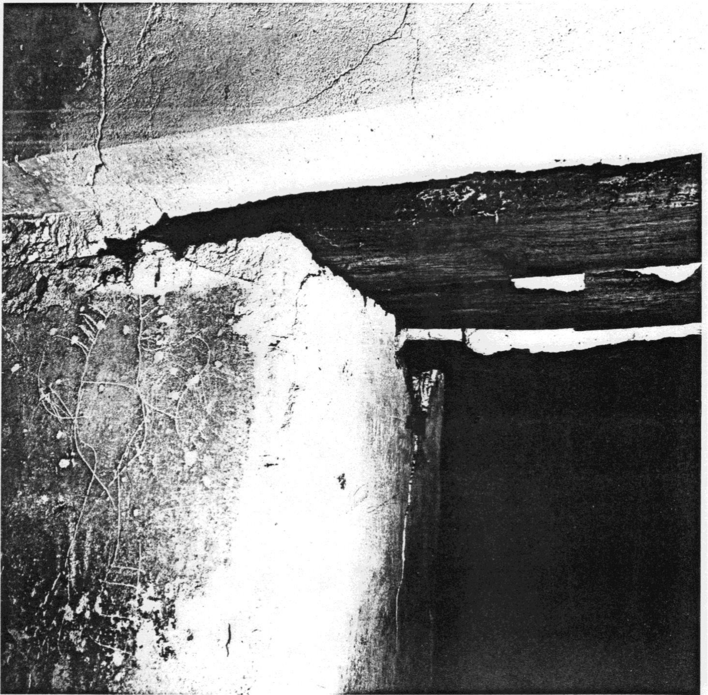
Fig. 5. Santa Rosa Xtampak, Main Palace, west side, inner room (24 or 26, Andrews' 1988 numeration). The wall plaster is still in amazing original condition. The degree of shrinkage can be measured as the distance the wood has retreated from the plaster; the plaster forms a mold of the wood at its original 7th-9th century size.
