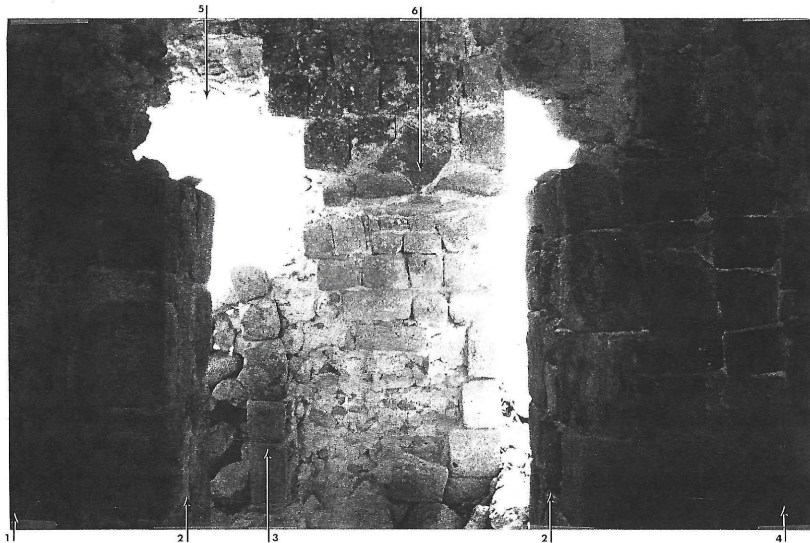
Fig. 21 - Looking west from inside Rm-#5, through Drwy-#1, into Pass-#2, then through Pass-1 to the outside (plaza), (1) south/west corner of Rm-#5, (2) jambs of Drwy-#1, (3) north-jamb of Drwy-#2 (with upper corner stones collapsing), (4) north/west corner of Rm-#5, (5) collapse above Drwy-#2, (6) only place where plaster covers medial-molding.
