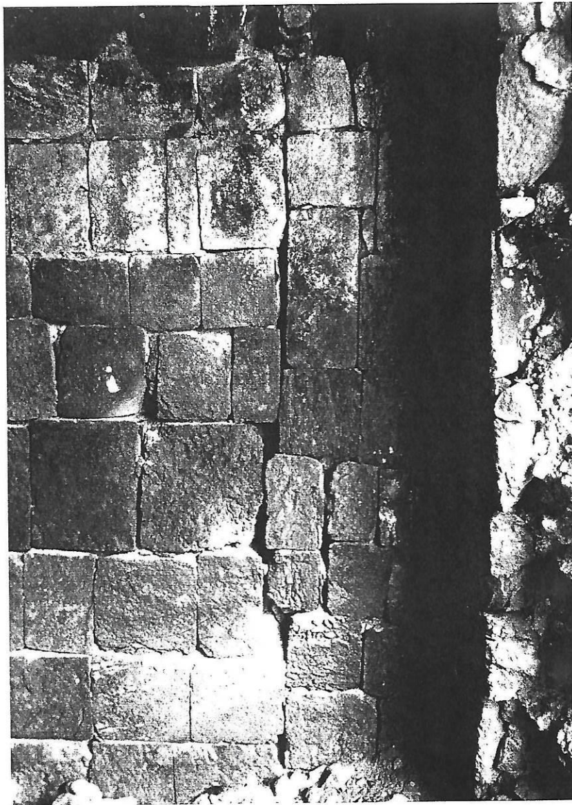
Fig. 7b - ROOM-#5, east-end of north-wall, showing roughly vertical line (starting just below a pair of "cross-beam" sockets) - original wall courses, on left, altered ones on right.
