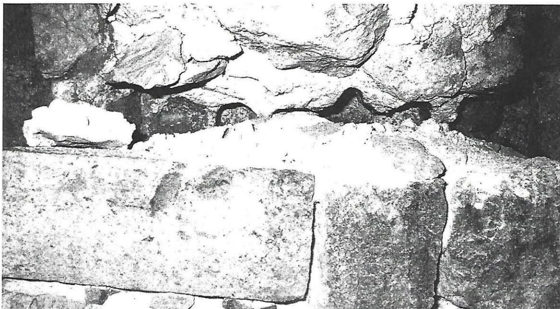
Fig. 11a - Looking directly at the north jamb of Drwy-#1 showing some of the "molds" of a lintel made of "poles."
