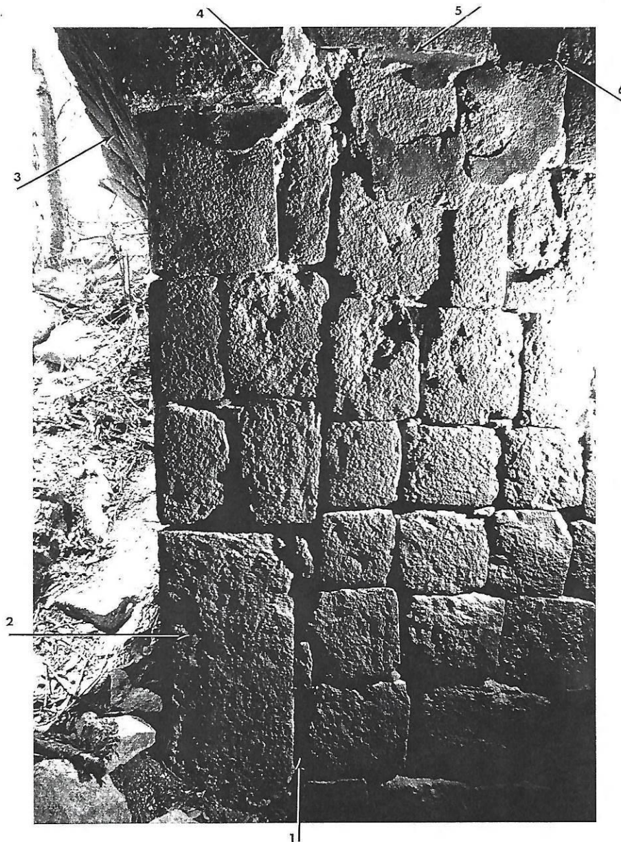
Fig. 7c - ROOM-#5, east end of South-Wall, showing vertical line in masonry (1) at what would be the approximate intersecting point with the east end-wall, (2) large jamb-stone at corner, (3) remains of the west vault of Pass-#3, (4) unusual "join" of Pass-#3 vault-spring as it jogs up, to meet the (higher) Rm-#5 vault-spring (see also Fig. 10b), (5) offset vault-spring of the south-wall of Rm#5, (6) left-most, of a pair of cross-beam sockets.
