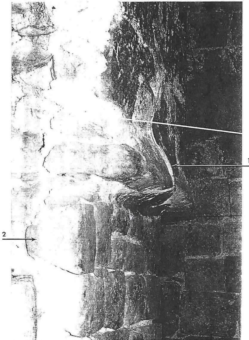
Fig. 24 - Looking north in Pass-#2 (same view as Fig. 22) showing (1) plaster covering the medial molding, (2) deeply wedged veneer-stone. white "level-line" is shown in foreground.
