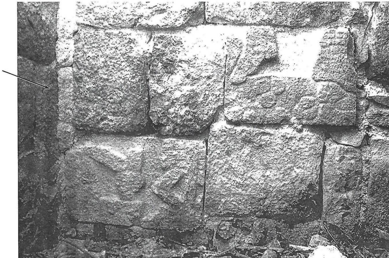
Fig. 33 - "REUSED-SCULPTED-STONES" used as interior-veneer, located in the west-wall of Pass-#2, in the south-west corner. One is "dancing" feet and the other seems to be part of a kings scepter or ceremonial spear. Veneer-stones of earlier construction (arrow) are seen going behind the west-wall.
