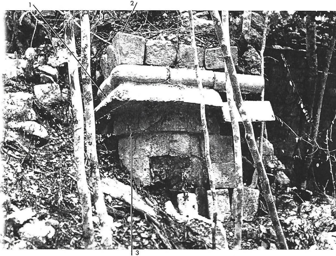
Fig. 14 - Large three-quarter-round end-column at north-end of Rm-#3 (south-wing of East-Range). Area to left is a predicted stairway - if so the corner of the building projects significantly out in front of the stairway. (1) unusual three-part medial-molding - lowest member is very sharply angled outward, also (2) upper corner piece angles upward, (3) collar at top of column.
