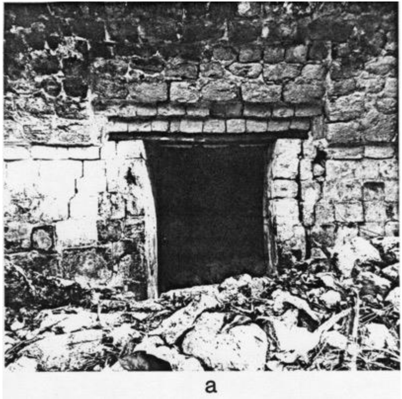
Figure 4, a. Front of Room 6 showing stepped recessed area over the lintel.
