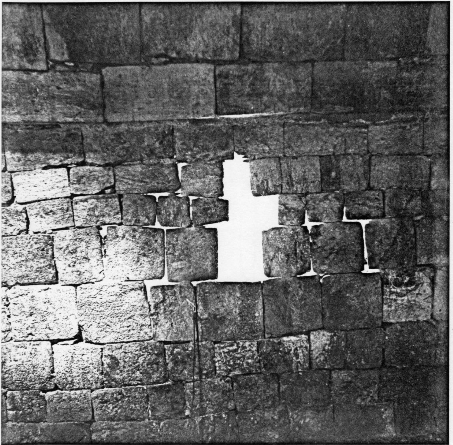
Plate 20. The west wall of Room 3 has crumbled about as far as possible without falling to ruin. The entire outside facade is gone, even the mortar between the stones of the inner facing. You can see right through the wall- (collapse in slow motion). Southwest Building. Unless this structure is repaired immediately these will be the last photographs--actually the only photographs since other expeditions were not equipped for interior photography.
