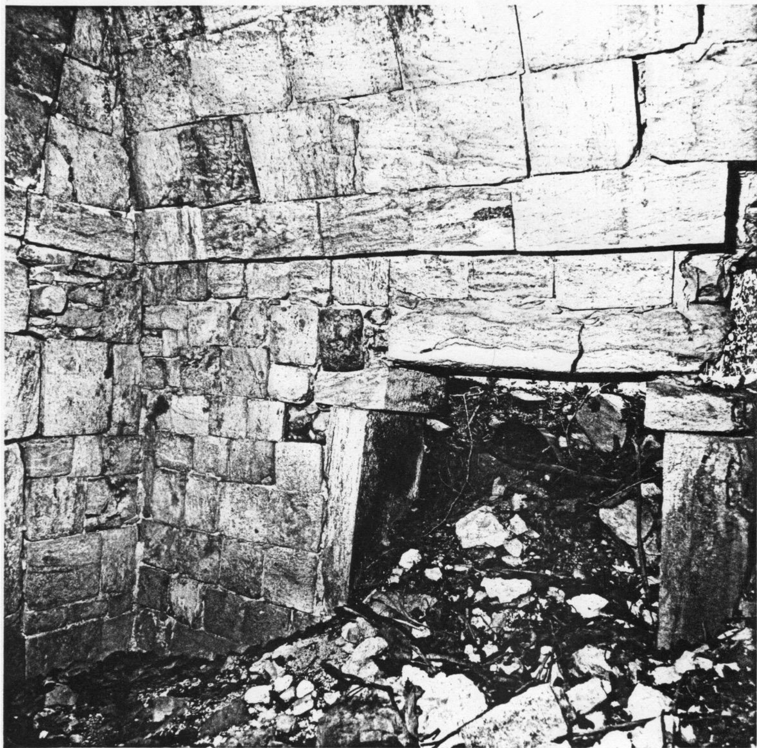
Plate 19. The front entrances of the lower rooms have half capitals on rectangular jambs; the inner doorways have no capitals at all. In the upper section the inner doorways have the half capitals—the front doorways are collapsed but may have been the location of the fallen column out in front. Inside Room 3 looking out. Southwest Building.
