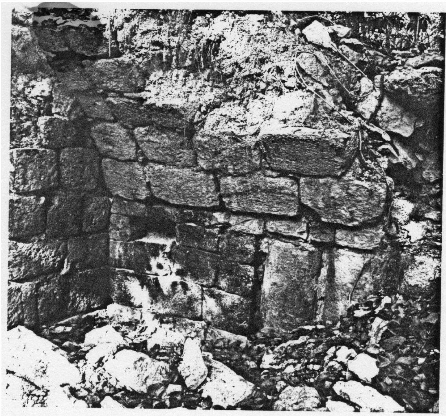
Plate 37. A rare incidence of embedded columns inside a room, in the remains of the East Range of the Cuartel. The stones directly above are of the vault soffit. The end wall (to the left) has no spring. No end wall in the Cuartel area has a Puuc spring.
