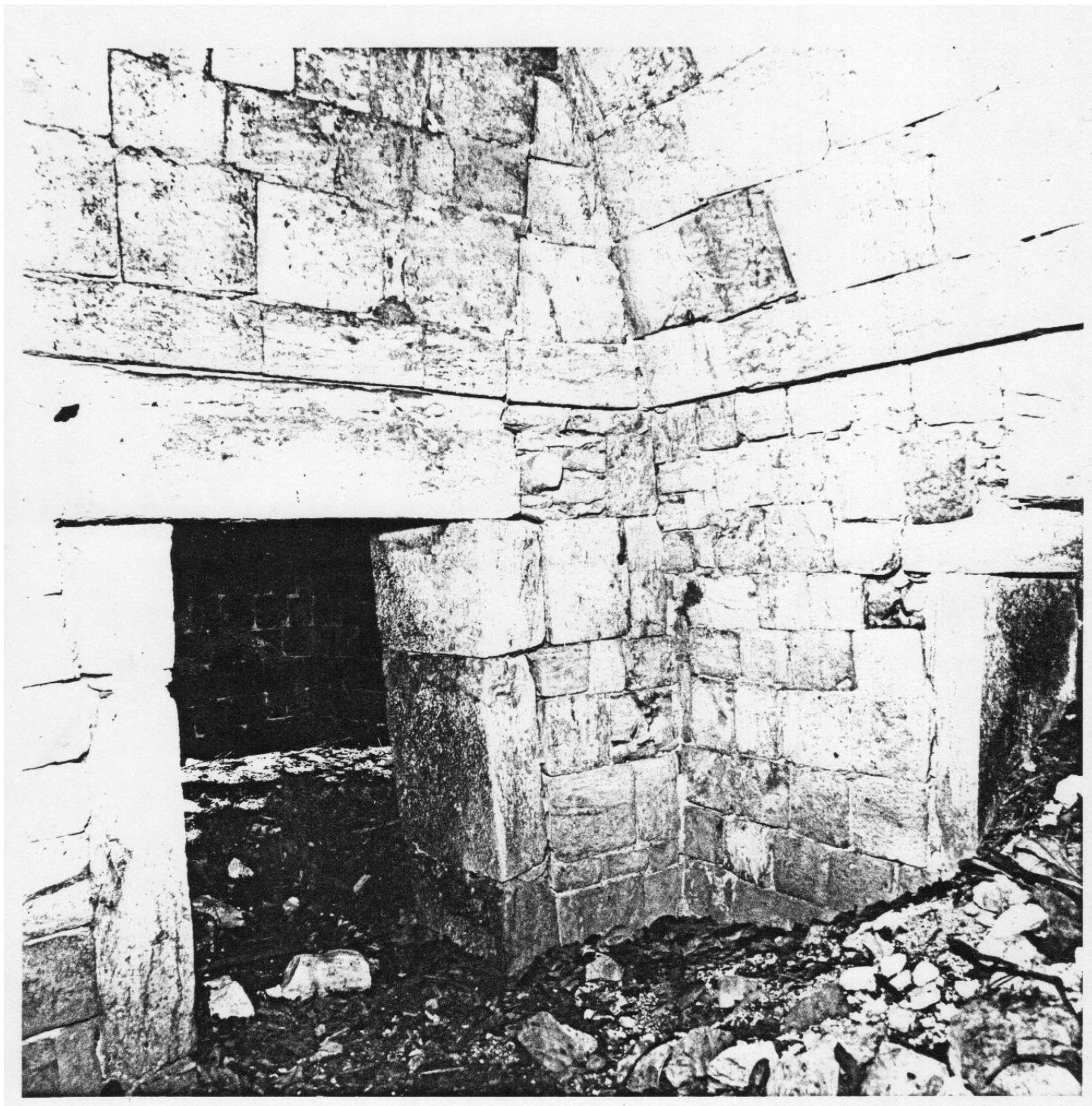
Fig. 4. Here is the standard for pure Puuc (at Xtampak at least)--yet we must also recognize that this would have changed over time. The finely squared vault stones are especially diagnostic of Puuc workmanship, as are the stone lintels and door jambs of monolithic size--the entire width of the door formed by a single stone (though almost always two or three stones high). Southwest Building, Room 3, looking east. 451608-12-Neg.13.
