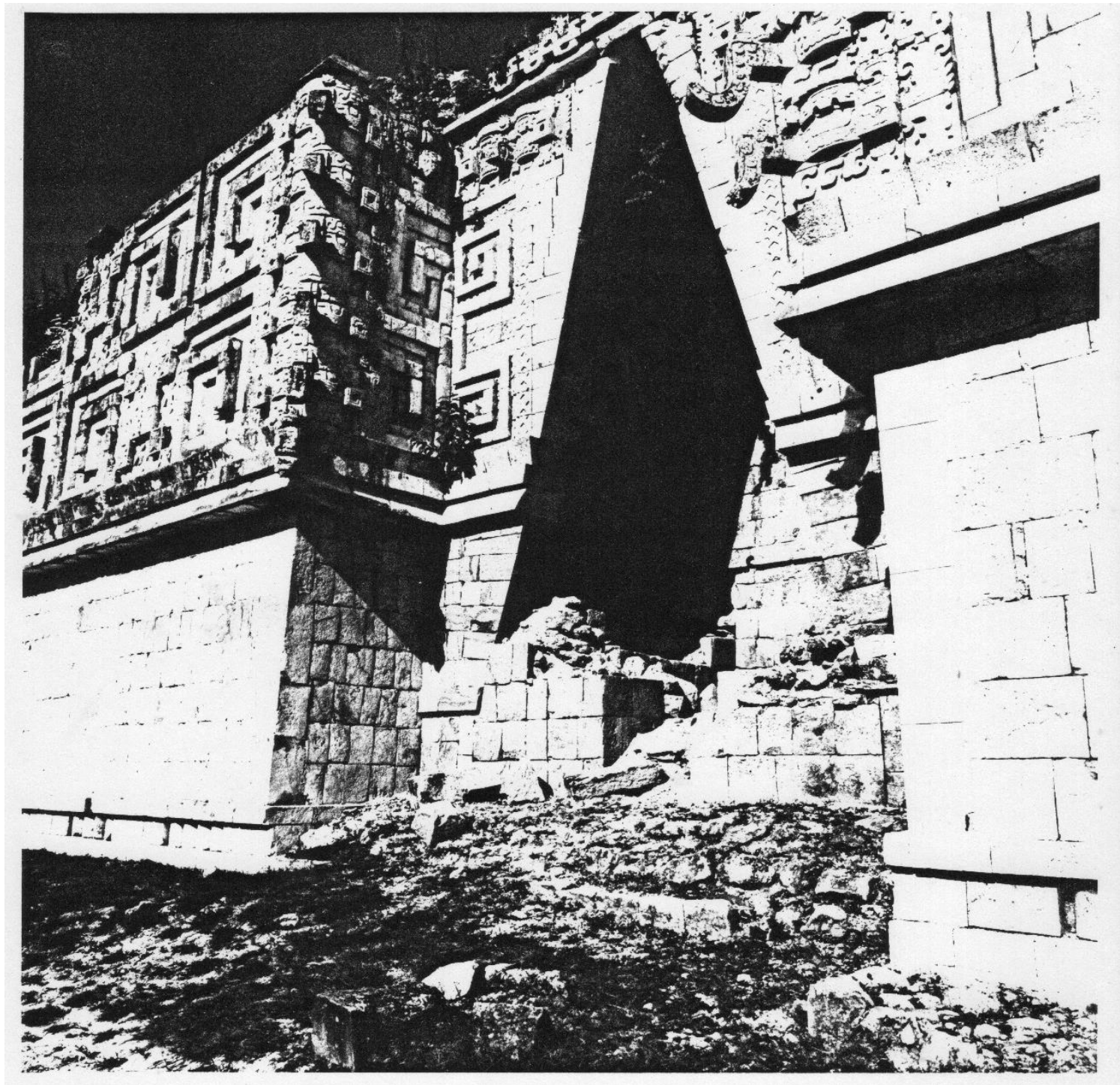
Fig. 5. The largest corbel-related vault yet known for any Puuc site. The corbel vaults in this building divide the structure visually into three units (though not noticeable in this close up view). Notice that the corner stones are of a specialized size and shape (corner in right foreground is restored but with proper sized stones). Uxmal, Palace of the Governors. 451608-6-Neg.16.
