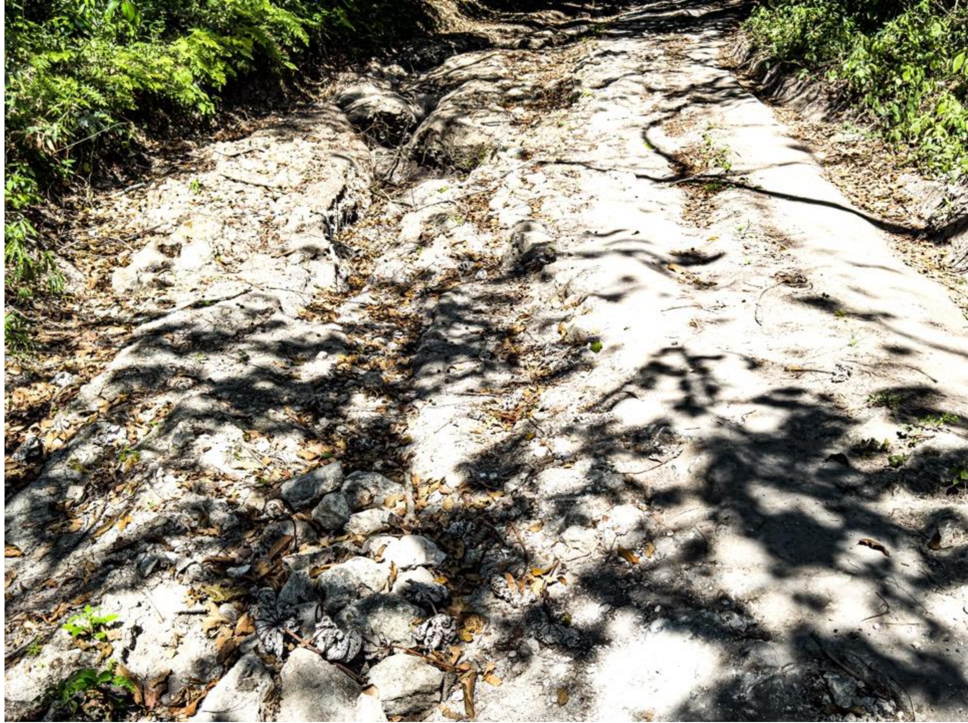
Fig. 69. The heavy rains of 2024 have completely washed out the sides of the road (as you can see at the top left).
