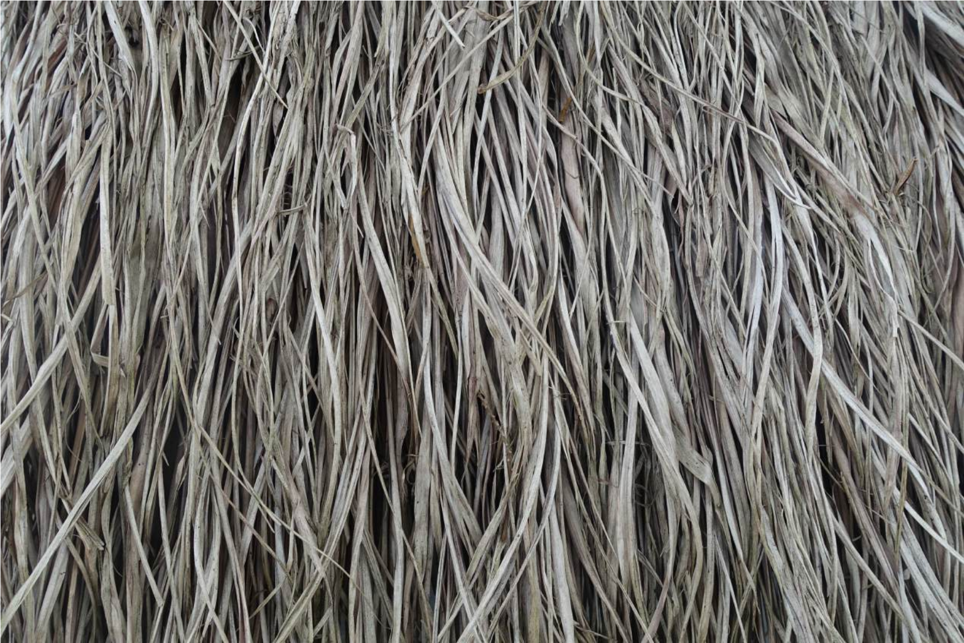
Closeup of roof thatch of ak grass
